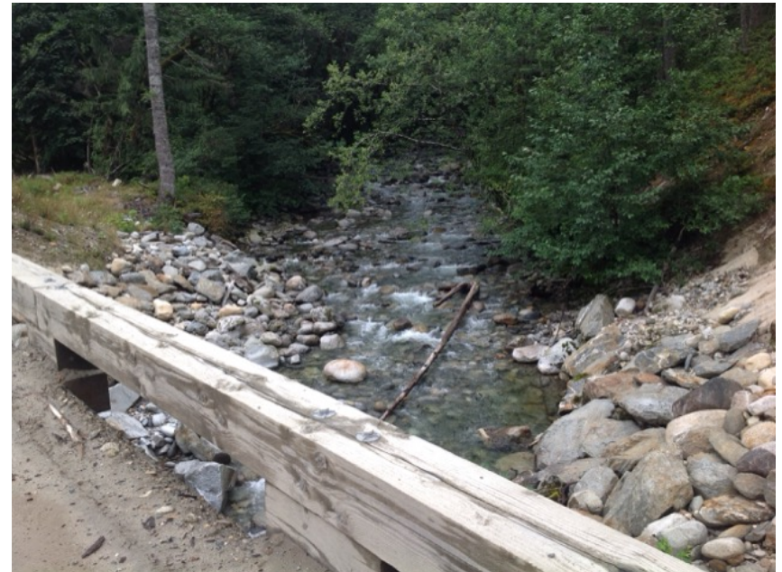
looking upstream from deck
