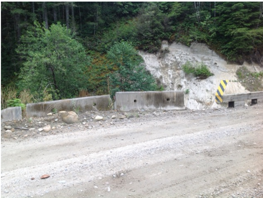
right bank upstream concrete no post barriers
