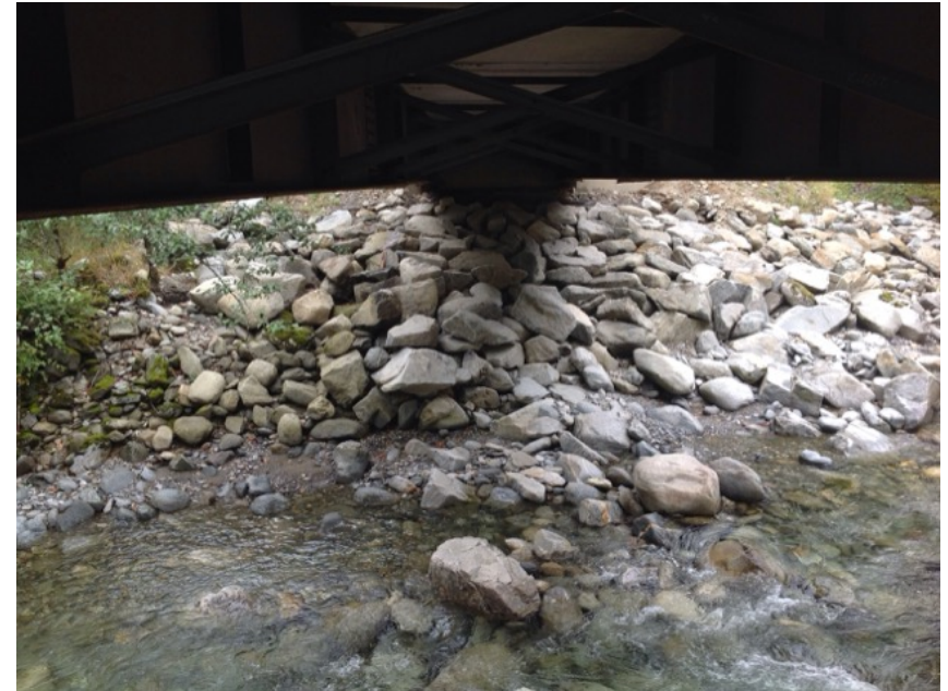
Right Bank Abutment when facing downstream
