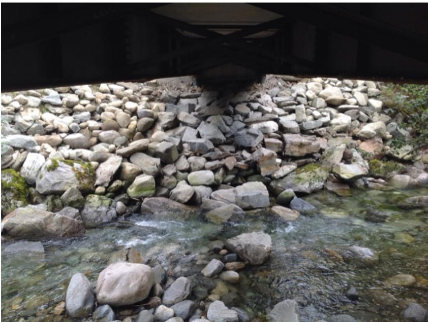
Left Bank Abutment when facing downstream
